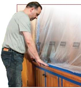
Norton masking tapes feature a special solvent-based, rubber adhesive system and strong holding properties. These tapes adhere and release cleanly while providing clean edges on a variety of flat, contoured, and irregular surfaces. Norton sheetings provides superior solvent, paint, and contaminant penetration resistance. Use them during paint preparation and anywhere you need work area protection. Tear-resistant properties allow movement without ripping.
